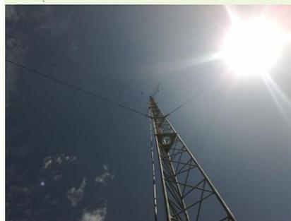
The wind monitoring masts and instruments are continually exposed to the harsh elements of our environment and must be inspected for wear. The masts are regularly checked and maintained by our in-house team of experts to make sure they remain in good operational condition.
