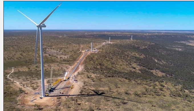
Hardstands - crane pad & equipment laydown area (blades, tower, nacelle etc.); 1.5 to 2 ha per turbine.
