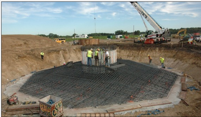
Tower foundations ~800m 3 concrete.
