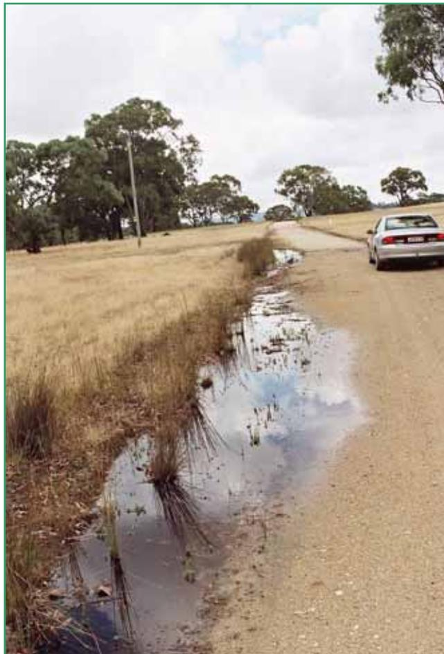
**Figure 3.4 Lerida Road North – water ponding.**
