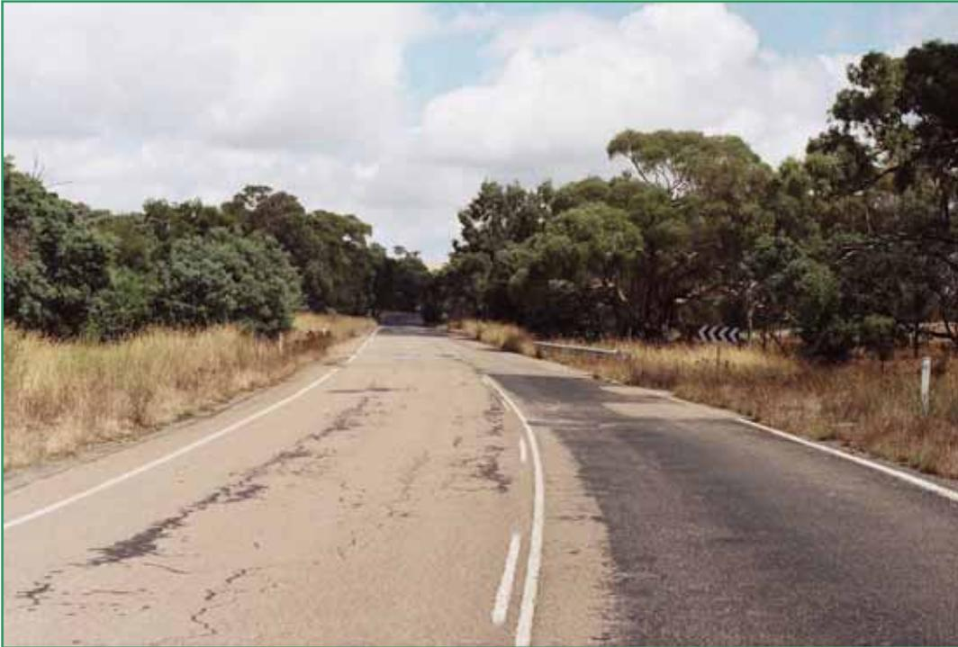
**Figure 3.6 Cullerin Road – pavement damage.**
